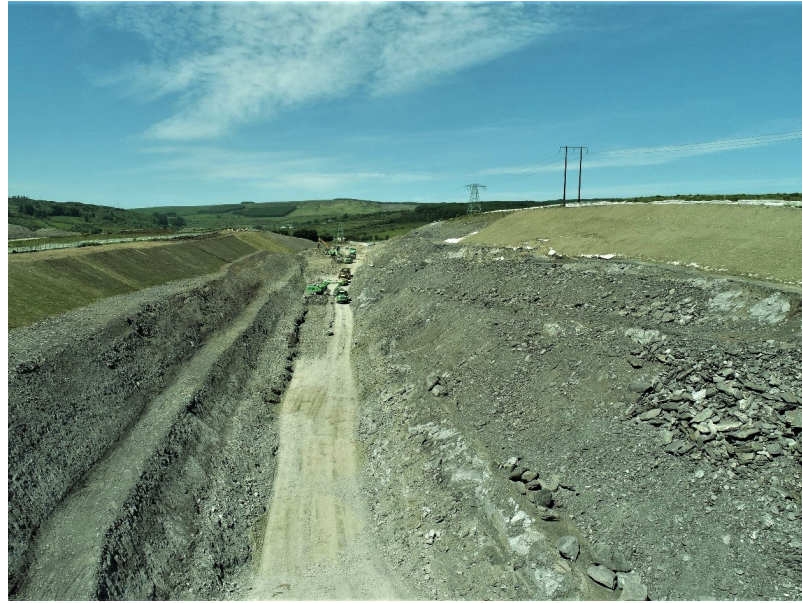
Rock Breaking & Bulk Excavation at Slievareagh
