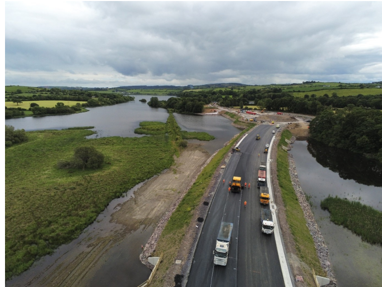
Roadbase Layer being laid from Coolcower Roundabout towards S25 Coolyhane Underbridge
