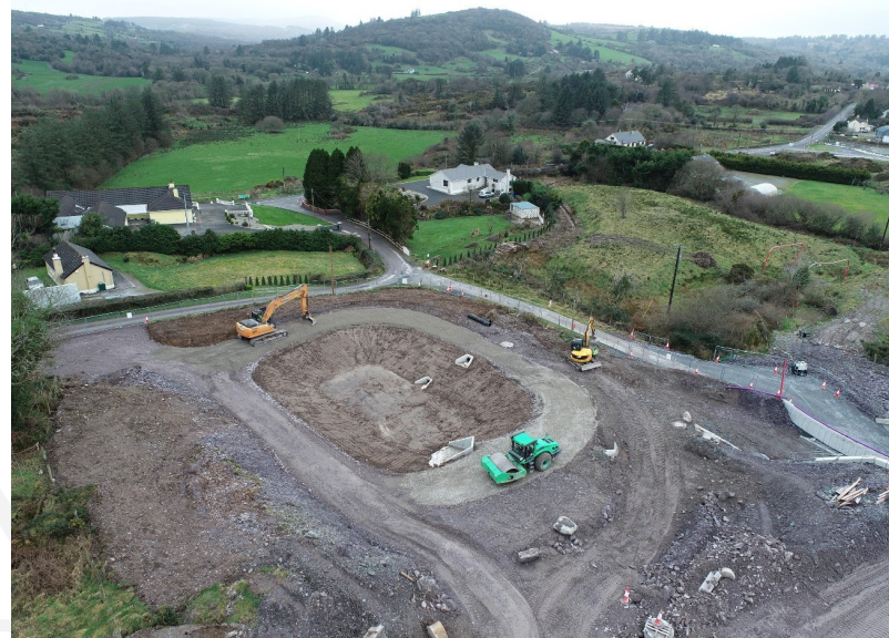
Completion of Attenuation Pond at Toonlane East
