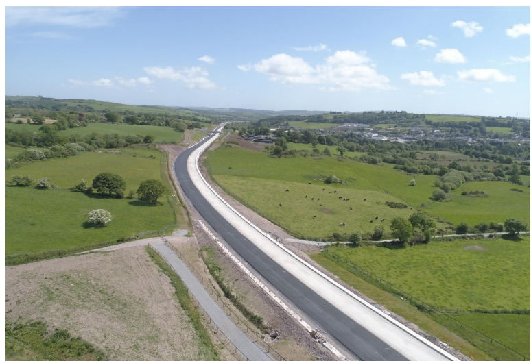
Roadbase Layer being laid at Ballyveerane
