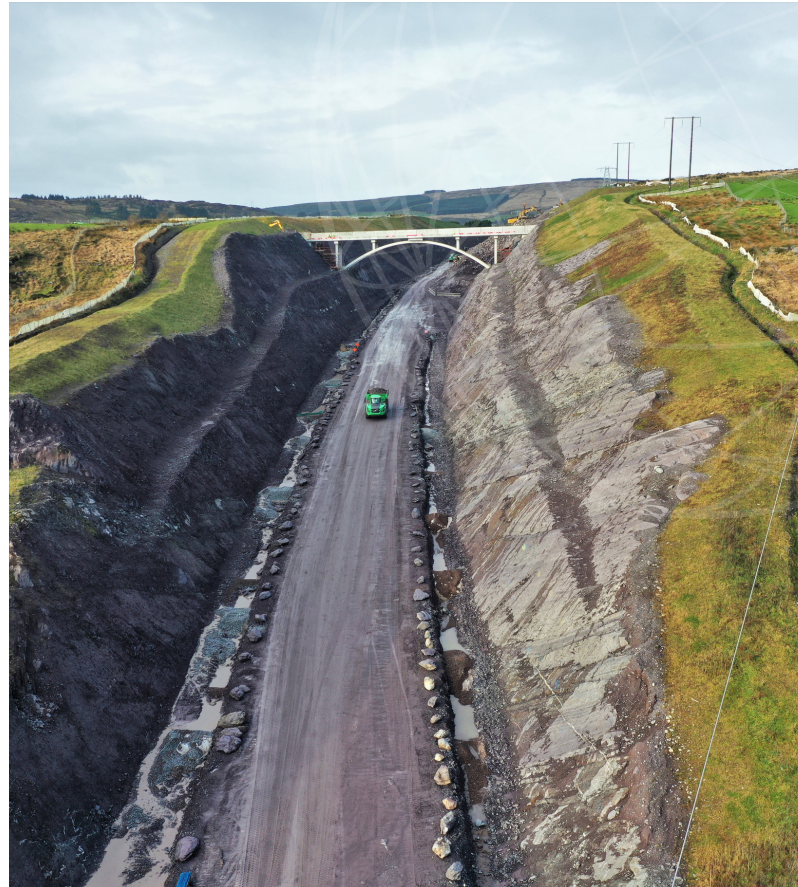
High level bridge at Slievareagh
