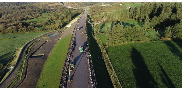
Drainage and ducting complete at Kippagh
