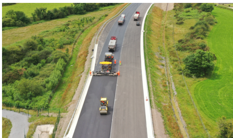
Wearing Course being laid at Cúil an Bhuacaigh
