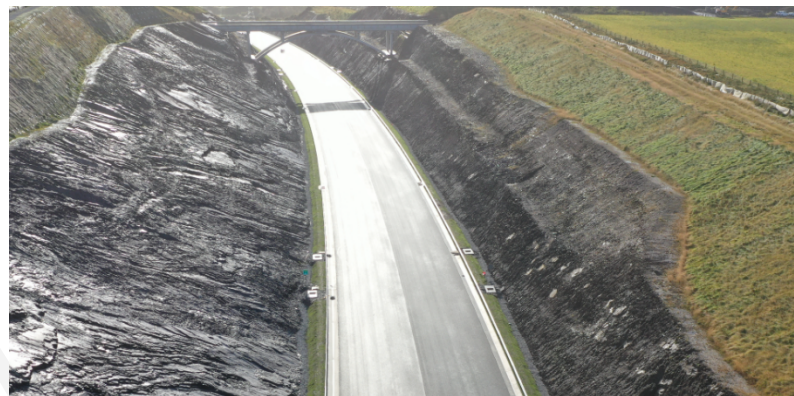
Wearing course complete at Cut 1
