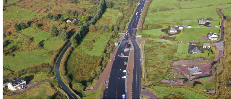
Temporary layout at Western Tie-In
