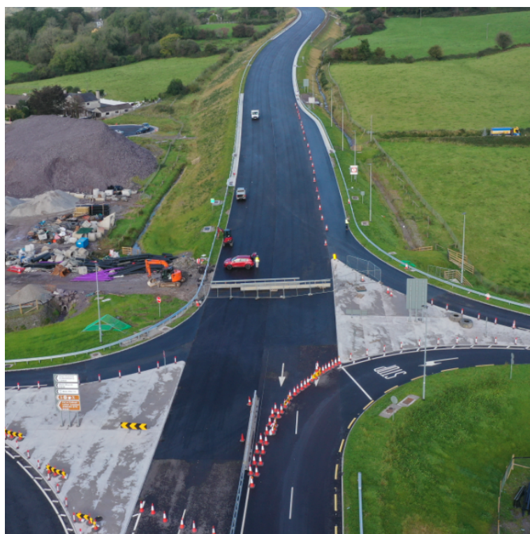
Toonlane traffic islands looking West
